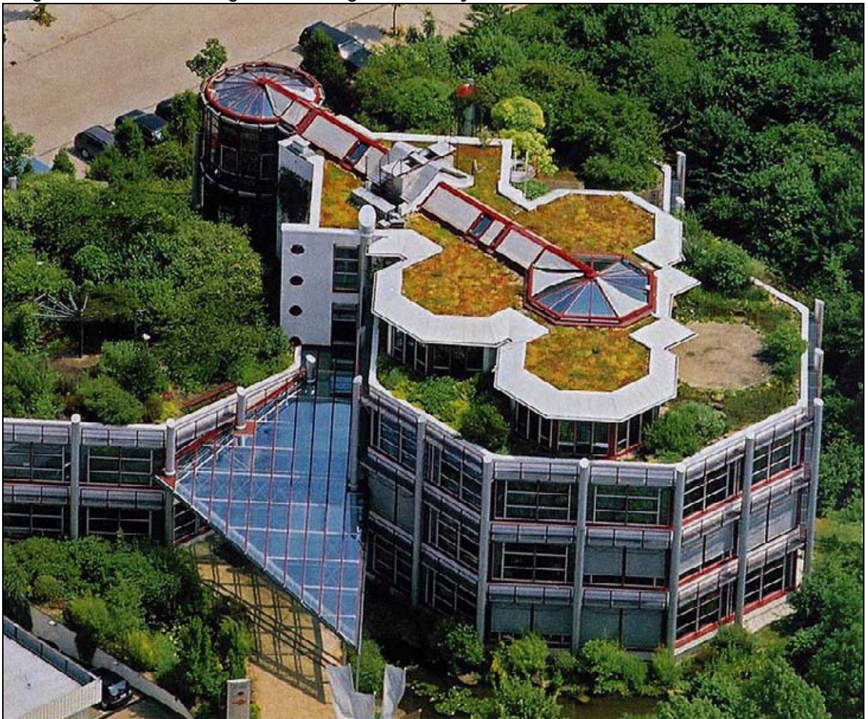
The building with its green roof level, eight years after completion, showing both intensive and extensive green roof systems. (Source and copyright © 2002 by Zinco Ltd.)
