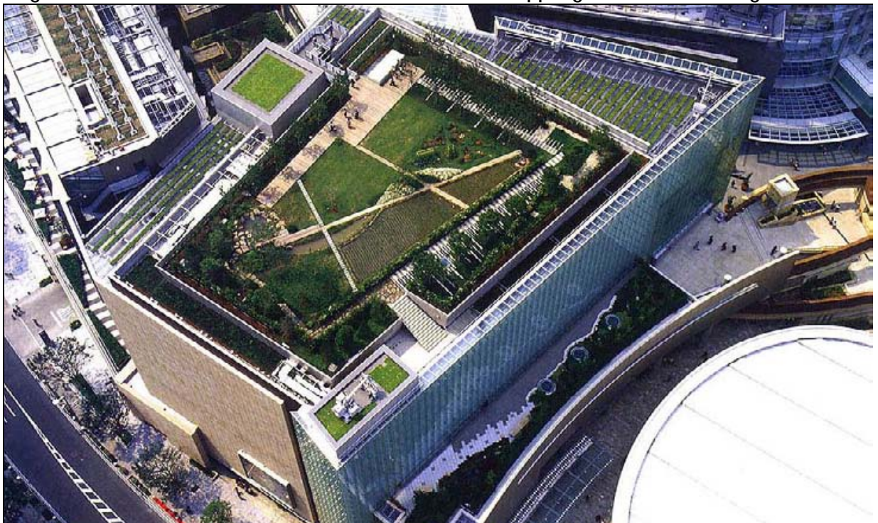
This green roof includes intensive and extensive green roofs, arranged so that the public space is not obstructed by utilities. (Source and copyright © Earth Pledge, 2005)
