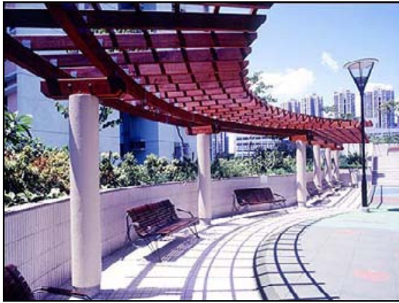
16.2 – Fanling Departmental Quarter (North District) (Source and copyright © by ArchSD)
