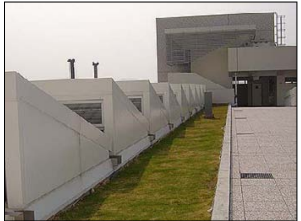
18.2 – Prim School, Area 65, Tseung Kwan O (Sai Kung District) (Source and copyright © by ArchSD)
